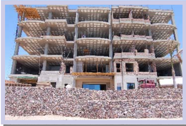
Right: View of Building A from the San Francisco Beach.
