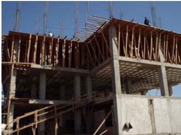
Left: Concrete being poured for the fourth floor of Building A.
