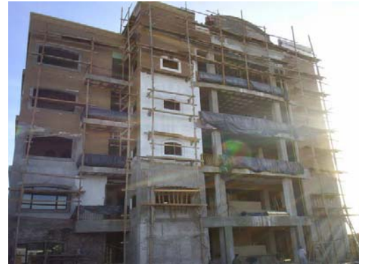
Above: Street-side view of Building A.
